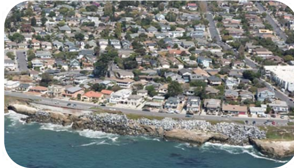
West Cliff Drive, Santa Cruz (Coastal Records Project, 2015)
